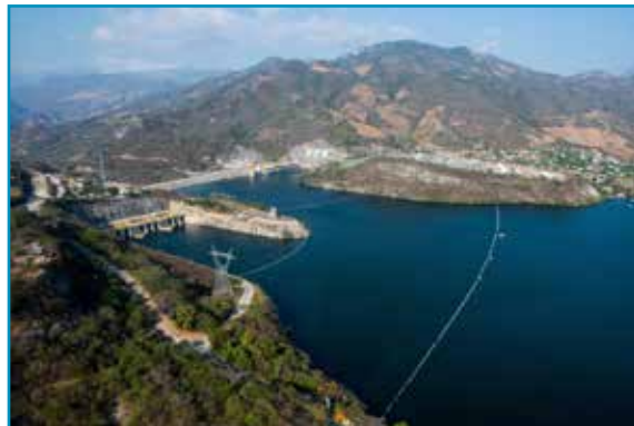
Hydroelectric power station Chicoasén, Chiapas.
