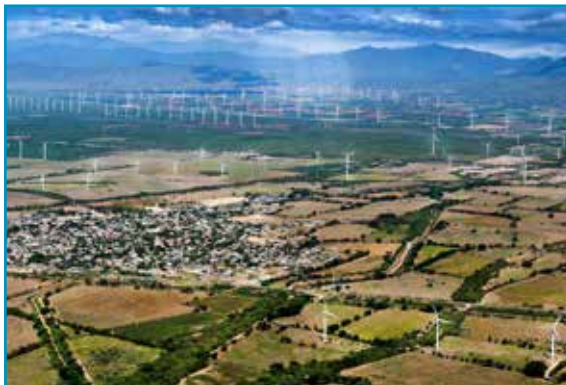
Wind power plant in La Ventosa, Oaxaca.
